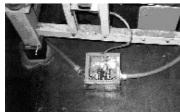
Conductors must be protected from abrasion.
